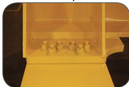
Standard bolted girder connection plates
